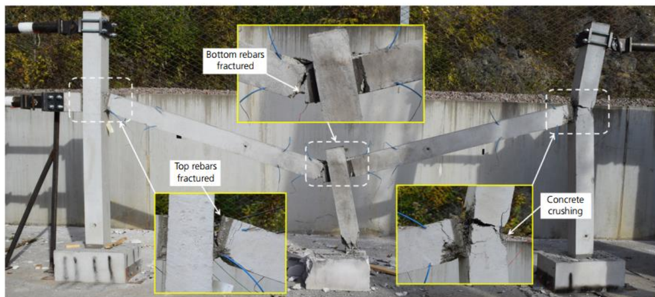
Fig. 7. General view of the failure of reinforced concrete frame elements in the study by Pham et al. [15]
